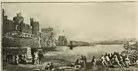
BUILDING THE CONWAY BRIDGE.
